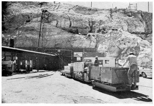
ENTRANCE to a tunnel site prior to an underground test is scene of massed activity as miners shuttle equipment into the tunnel and engineers check cables and instrumentation. Large pipe leading into the tunnel is part of the Sandia-designed air filtration system.
